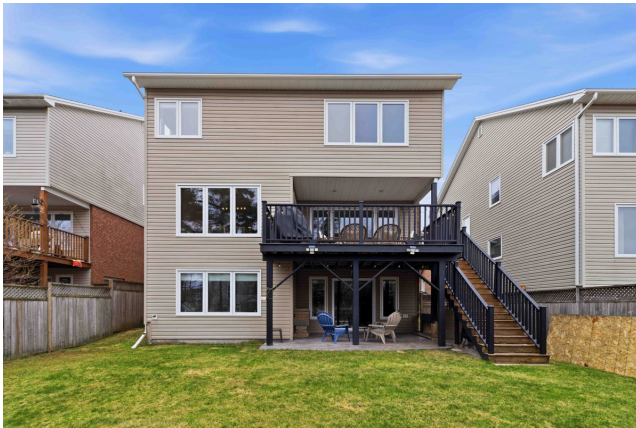
Back of house with deck and patio
