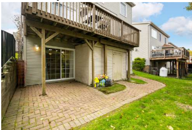
Good-sized shed under the deck
