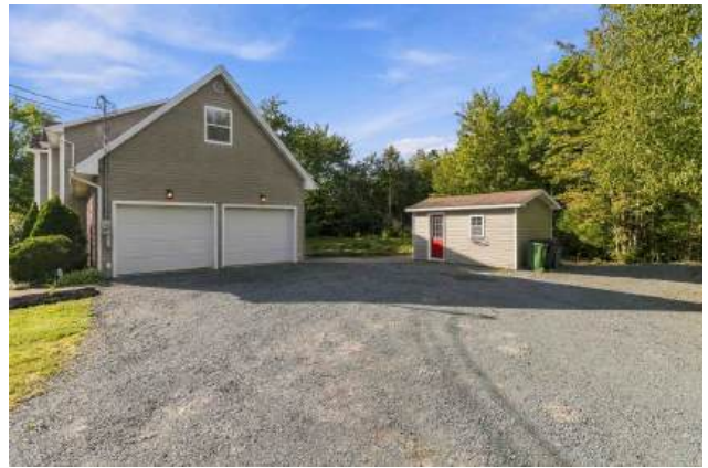
Double attached garage & Graves Barns shed
